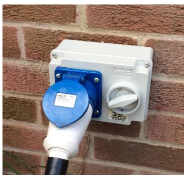
Figure 6 – 32amp Ceeform plug & socket
