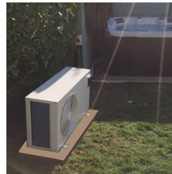
Figure 10 – Heat Pump Base
